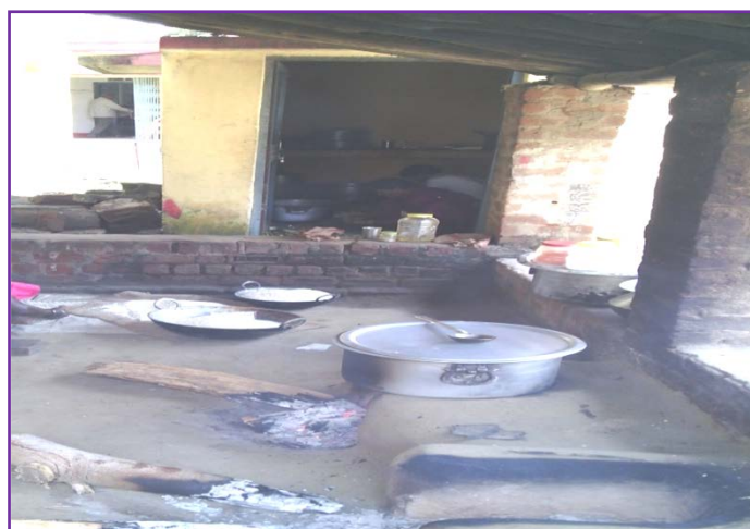
Kitchen shed in sample school
